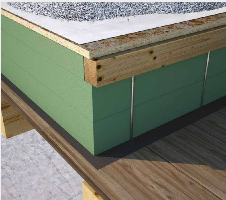
^ Fastening of hard insulation on a flat roof.
