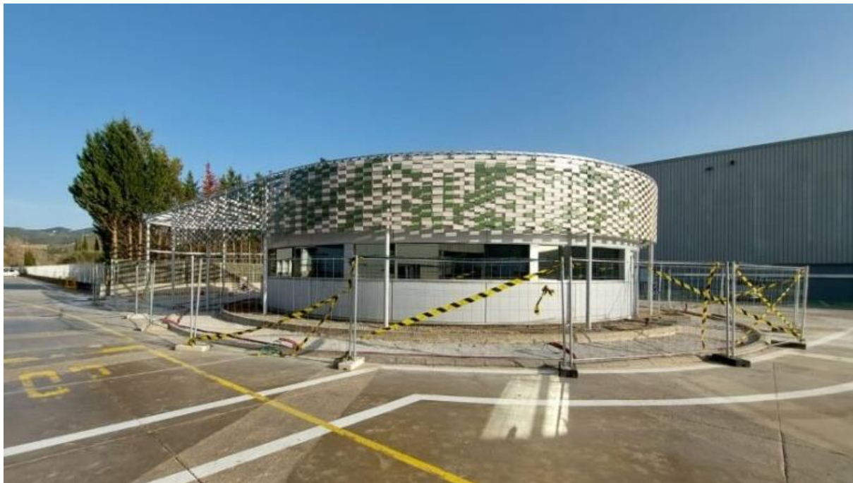
Figure 27 Control building in Sant Sadurn d'Anoia with partly installed integrated PV in an interwoven steel wire mesh – Living lab no. 24
