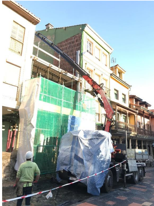
Figure 22: Construction site in Aviles, Spain in October 2023 – Living lab no. 8
