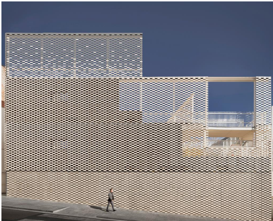
Figure 24: Kindergarten and primary school before renovation in Barcelona, Spain – Living lab no. 18
