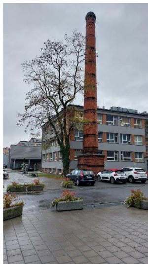
Figure 29 Historical chimney in the complex of Cracow University of Technology in Cracow – Living lab no. 26
