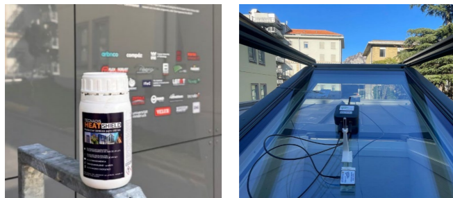
Application of the product within the BEEpilot test facility
